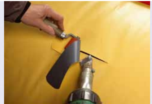
Hot air welded repair.
